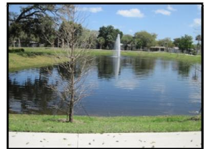
The pond also provided an attractive water feature for a passive park constructed on the premises. With proper maintenance, this wet detention system will provide much needed relief from nutrient loading in the Halifax River and will provide a closer step for South Daytona to achieve TMDL requirements of its surface waters.
