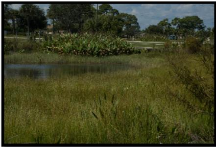
The stormwater strategy for this project was reduction of suspended solids and nutrients from runoff using BMPs to trap sediment and remove nutrients. This project includes the implementation of stormwater treatment BMPs, including the construction of nutrient separating baffle boxes, wet detention expansion (lake reconfiguration), swales, and filter marshes, which are all designed to reduce total suspended solids and nutrients.
