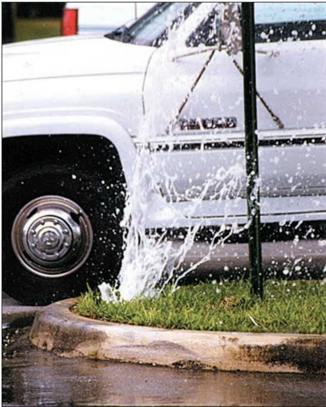
Figure 11. Water gushing from broken head.
