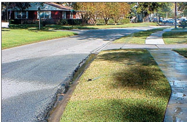
Figure 7. Poor design; sprinkler does not match area.
