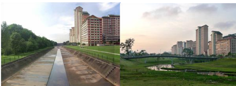
Figure 21. Before (left) and after (right) a stormwater infrastructure retrofit to establish Bishan-Ang Mo Kio Park in Singapore (images from PUB 2016).
