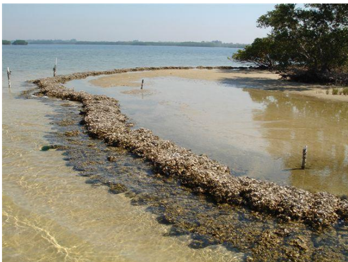
Figure 31. Oyster bag reef placed along the shoreline of Whiskey Stump Key.
