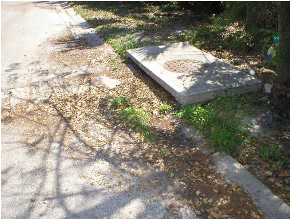
Figure 9. CC3 - Inlet on west side of Captain Kidd Ave. in Basin B3. Note leaf loads.
