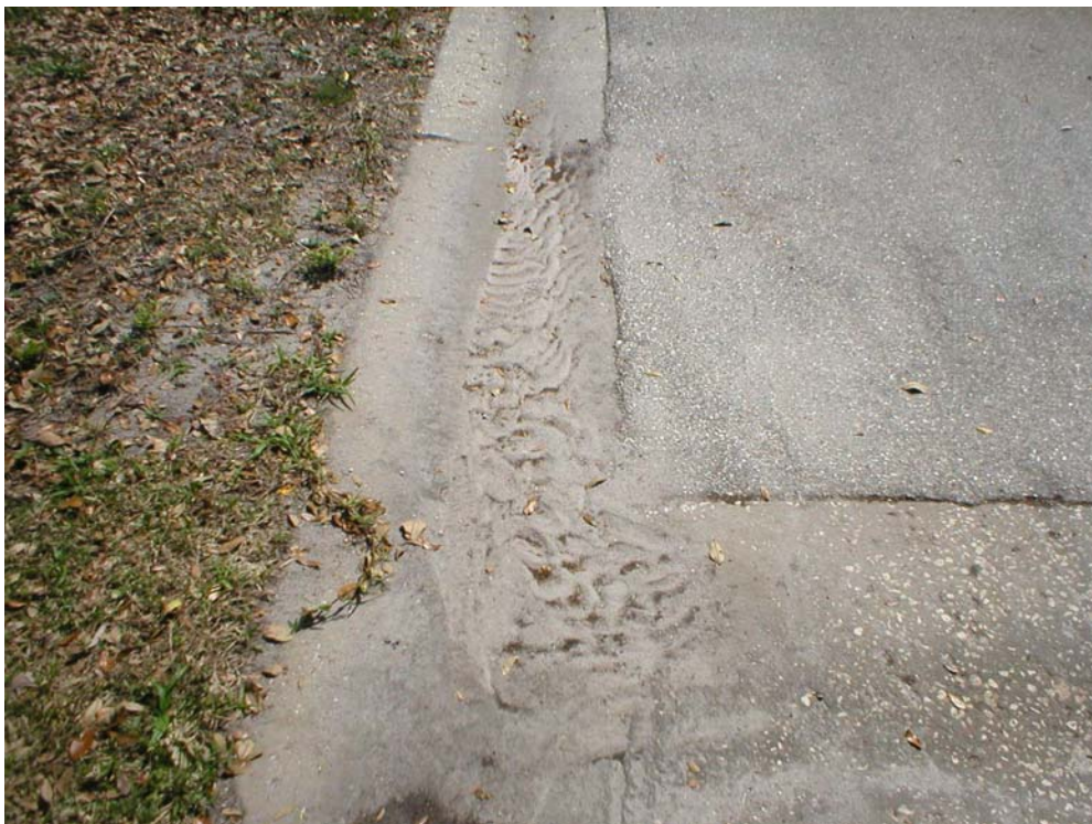
Figure 11. Sediment on curb across the street of outlet CC3.
