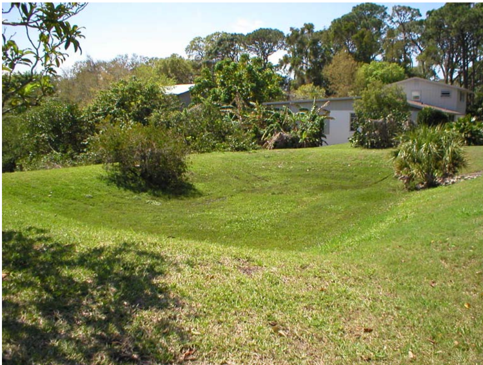
Figure 5. Dry Retention Pond upstream of outfall CC1.
