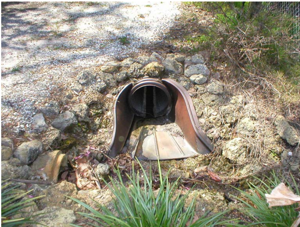
Figure 7. Outlet CC2 - mitered end on Captain Kidd Ave.
