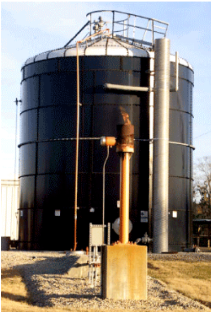
Fig. 12. Fixed-film anaerobic waste digester for methane production at the University of Florida. Photo courtesy of A. Wilkie.
