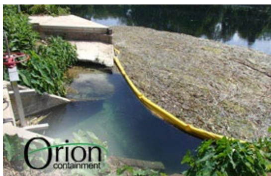
Example of Litter Collection System Containing Debris Source: Orion Containment 2019
