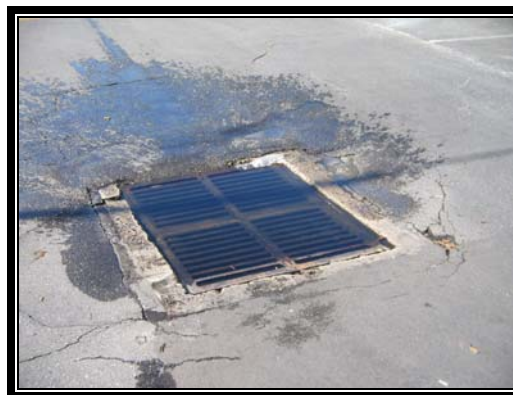
Photograph 35. This stormwater grate in the Fountain Bridge Apartment complex parking lot was consistently surcharged. Elevated bacteria concentrations and the human Bacteroides marker were detected in the water when sampled in December 2007 (station DHR10).
