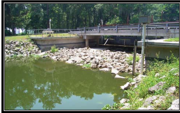
Photograph 11. Lake Thonotosassa control structure at the headwater of Flint Creek.
