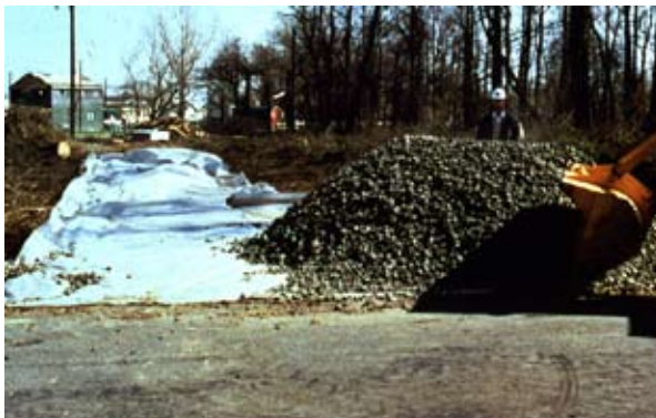
Stabilized construction entrance
