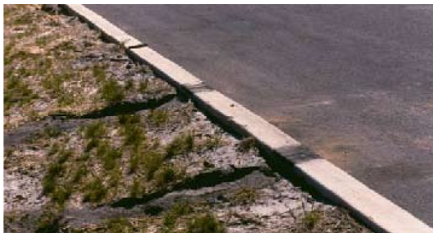
BAD: Lack of depressed curb hinders access to practice by maintenance personnel and equipment.
