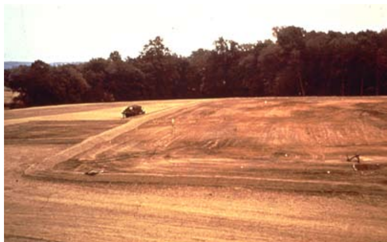
Example of an earth dike flow diversion
