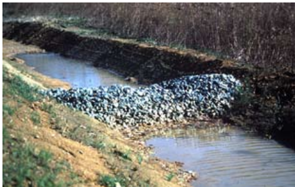
Examples of rock check dams
