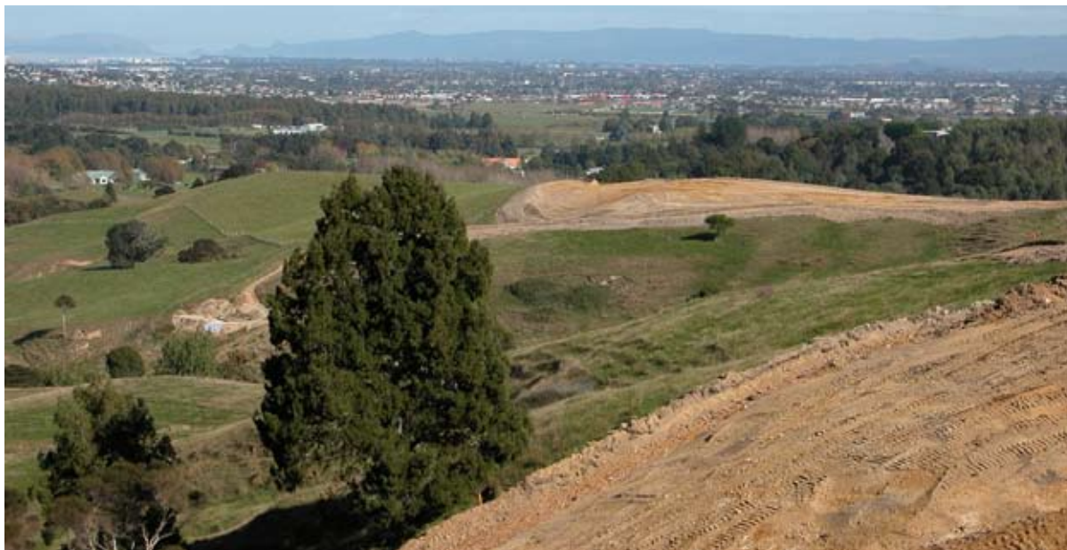
Minimal disturbance for earthmoving
