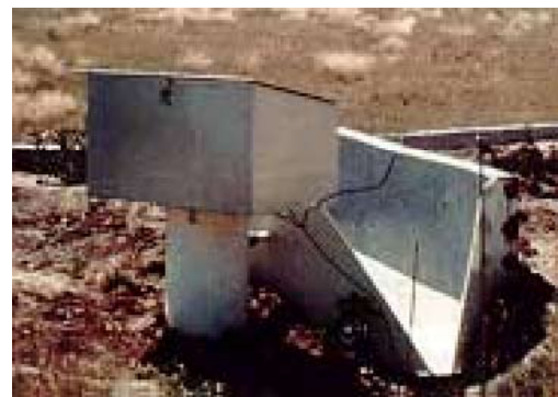
H-flume (with Instrument Shelter)
