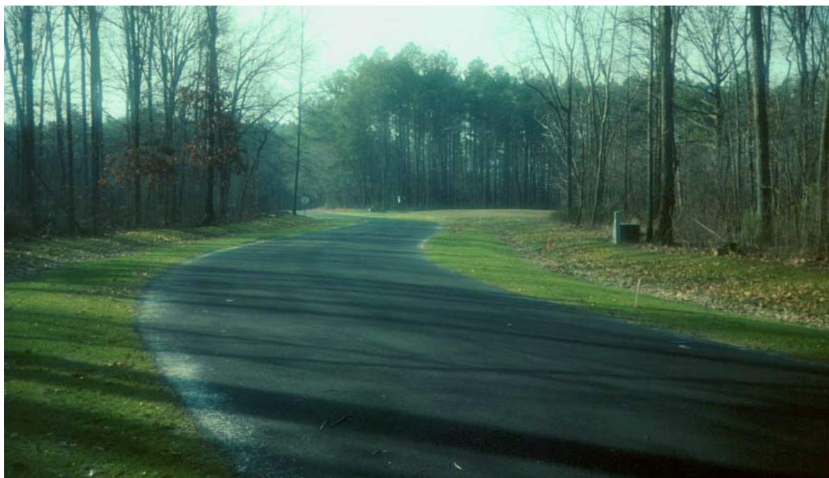
Subdivision without curbing or catch pits
