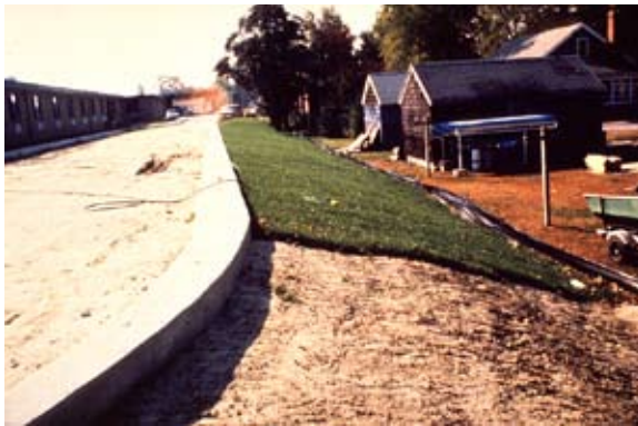
Turf being applied to topsoil
