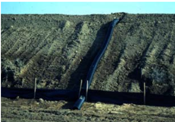
Examples of pipe and flume downdrains
