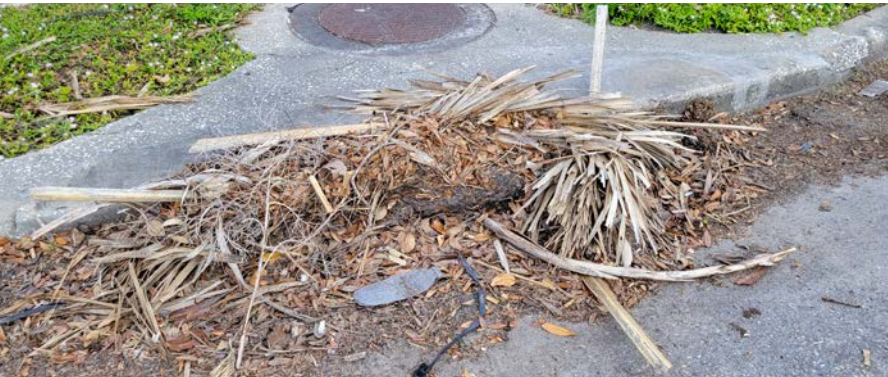
▲ Remove sediment and debris from stormdrains before they can clog pipes, cause flooding, or create sediment and litter problems in your pond | David Shafer.
