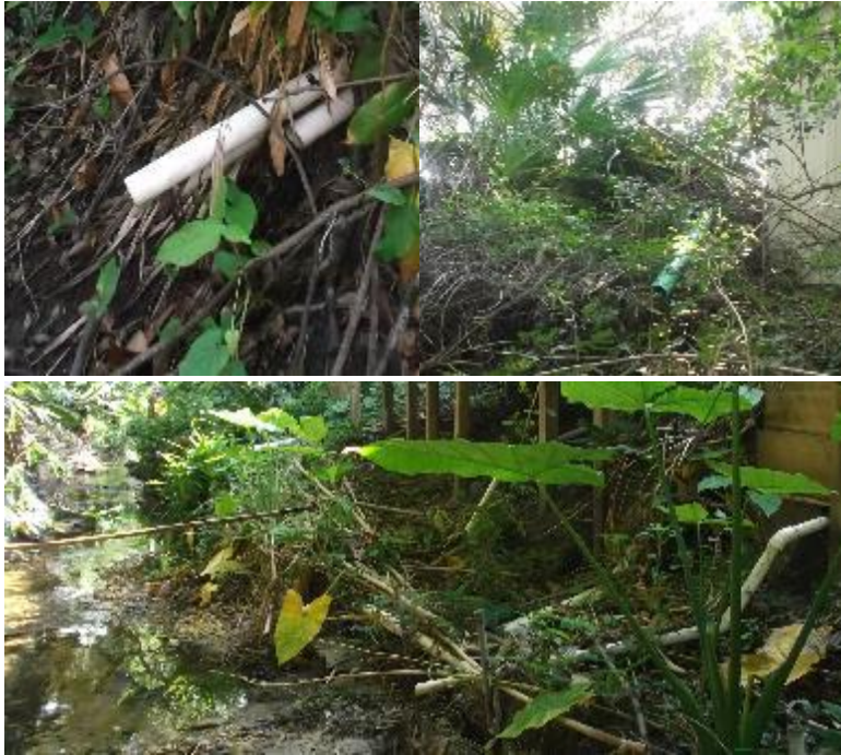
Figure 20. Illicit connections to Poinciana ditch
