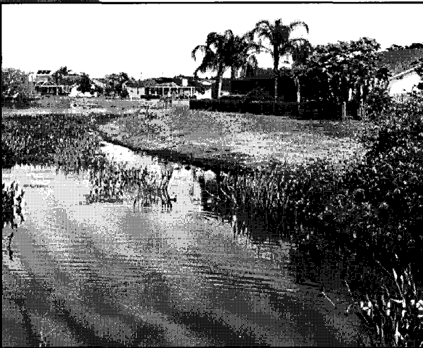
▲ Planted littoral zone in residential stormwater pond.
