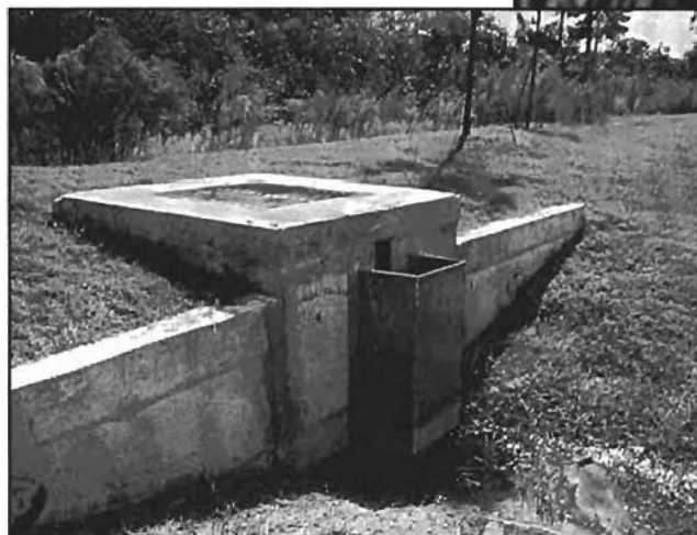
▲ Outflow Control Structure
