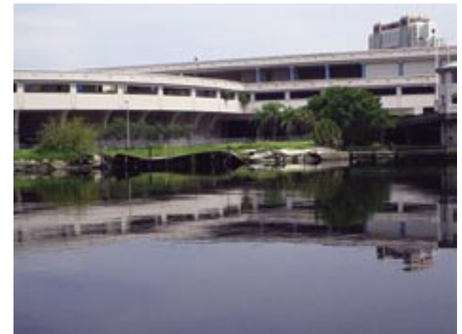
Figure 47: Rip-rapped shoreline with concrete rubble at Ribbon of Green Park.
